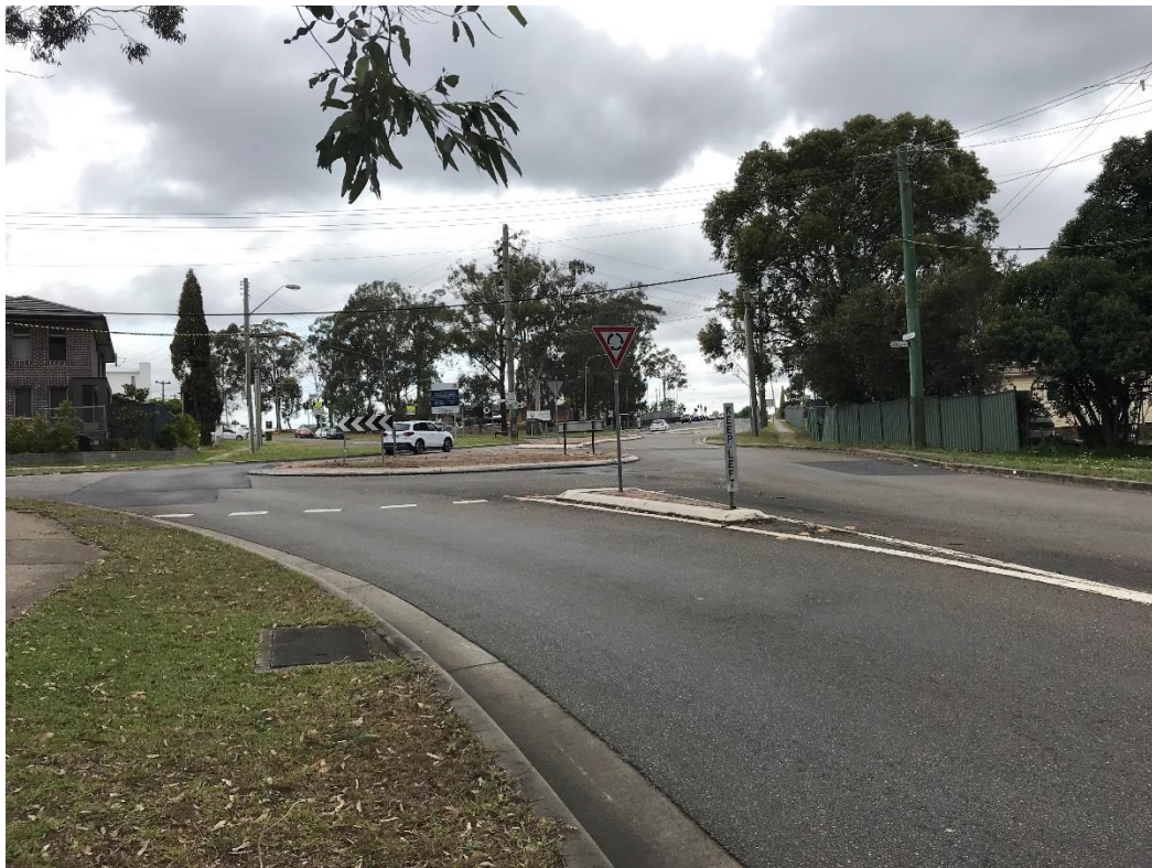
View looking south at the roundabout intersection of Blacktown Road and Metella Road
